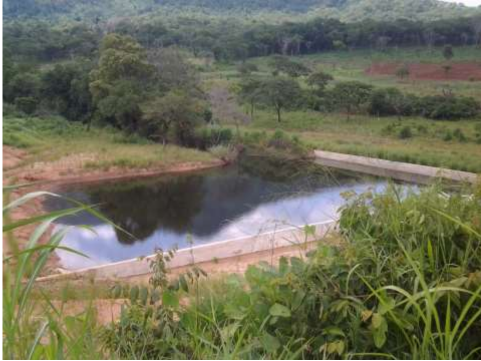
Figure 6-16-1: A typical PROIRRI/IRRIGA water retention infrastructure in Manica province
